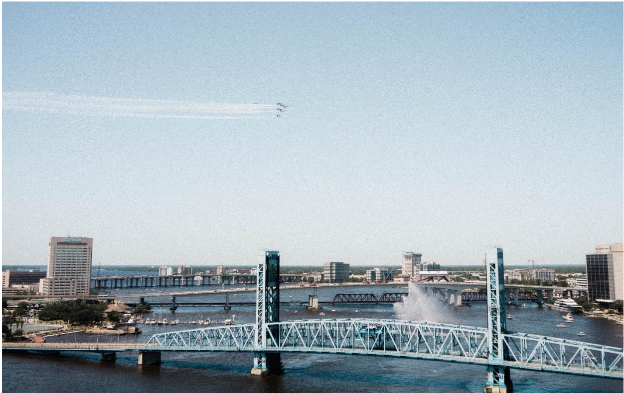
Figure 3-10. Flyover at St. Johns River
