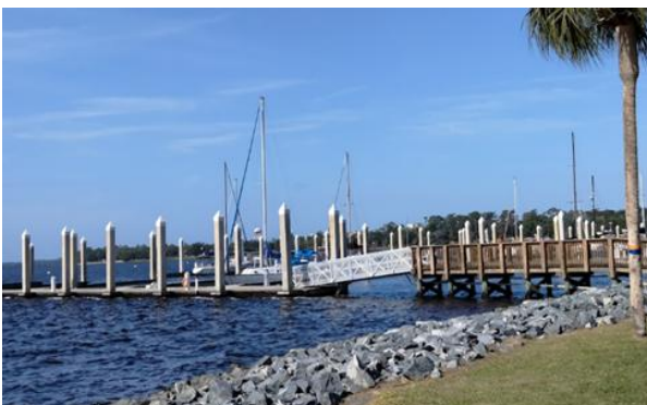
Figure 2-9C. Berm with Riprap along Mayport Shoreline
