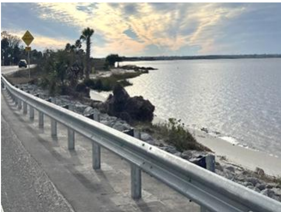
Figure 2-8C. Displaced Riprap along Mayport Shoreline
