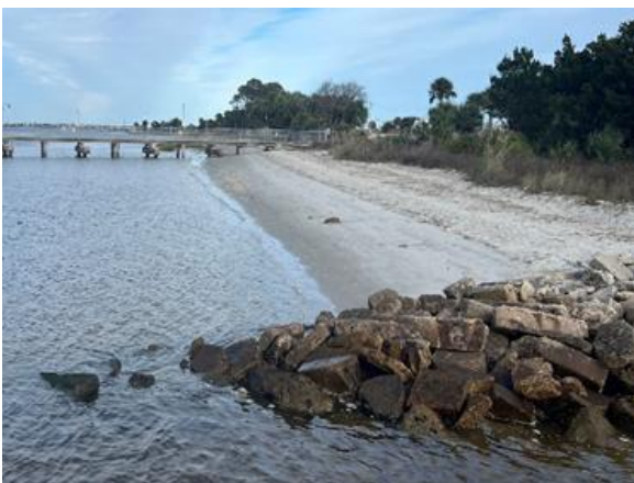
Figure 2-8C. Displaced Riprap along Mayport Shoreline
