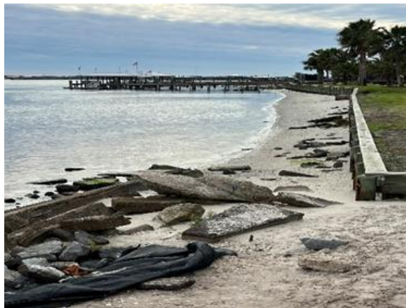
Figure 2-8D. Poorly Sorted, Aging Rip Rap along Mayport
