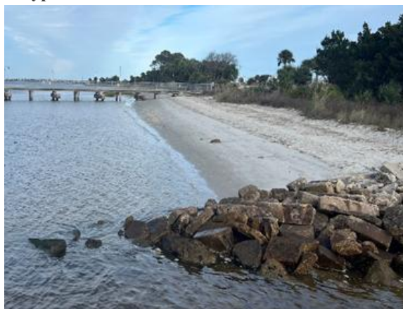
Figure 2-8D. Poorly Sorted, Aging Rip Rap along Mayport
