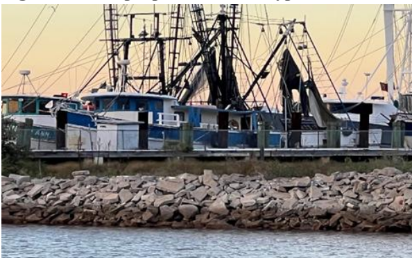
Figure 2-9C. Berm with Riprap along Mayport Shoreline
