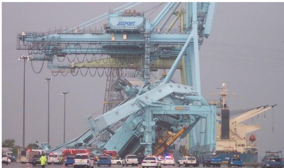
Figure 2-9. Aftermath of a Crane Collapse at the Jacksonville Port Authority (JAXPORT) Blount Island Marine Terminal on August 13, 2008, Following a Microburst Storm Event
